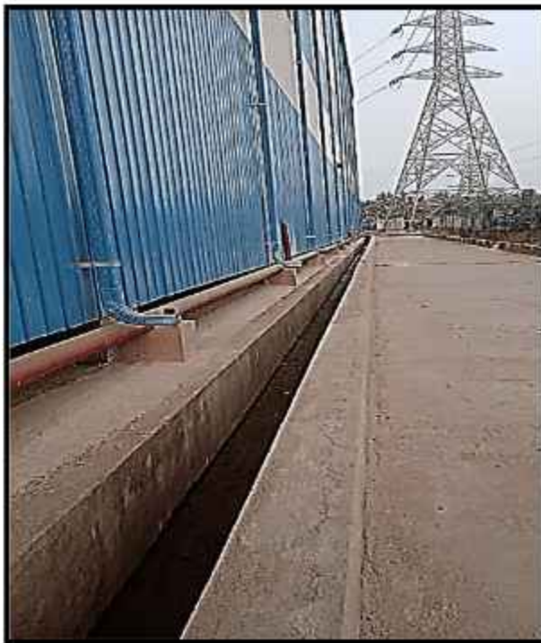
Connecting drain to Rain water Harvesting recharge pit nearstacker reclaimer
