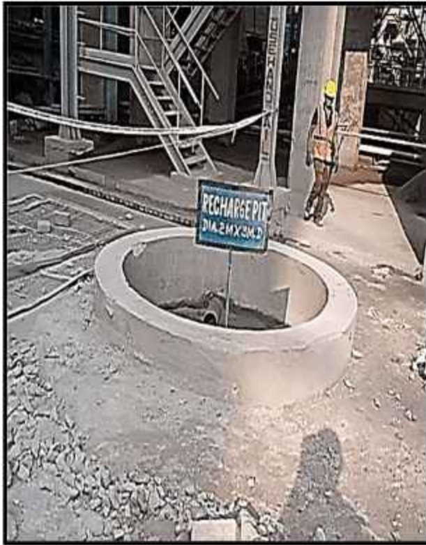
Rain Water Recharge Pit with connecting drain near mill area
