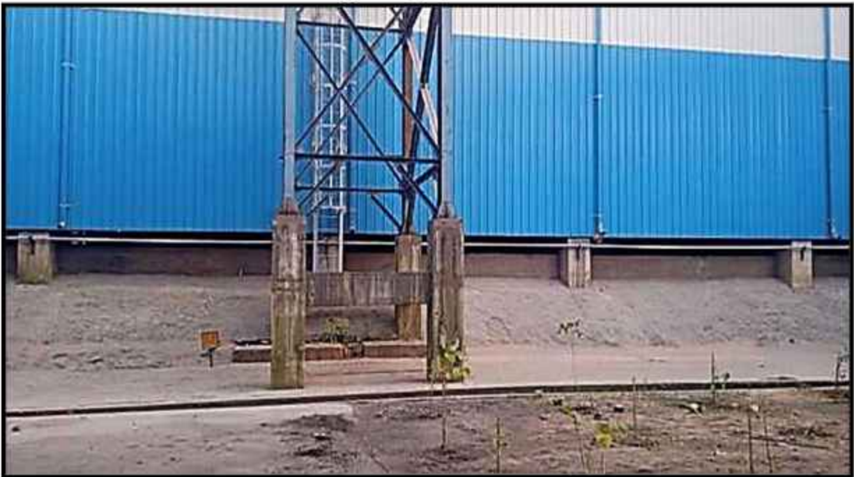
Rooftop Rain water collection pipe line, concreated drain connected to recharge pit near Electrical load center
