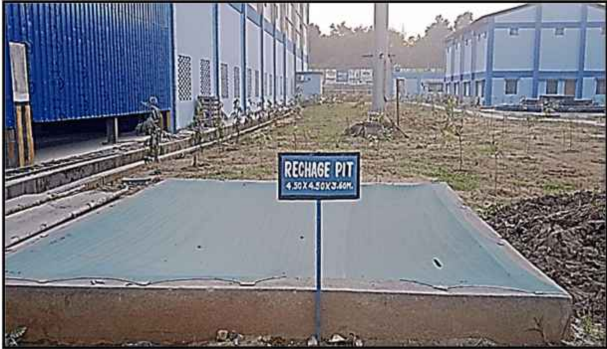
Rain water harvesting recharge pit near Packing plant
