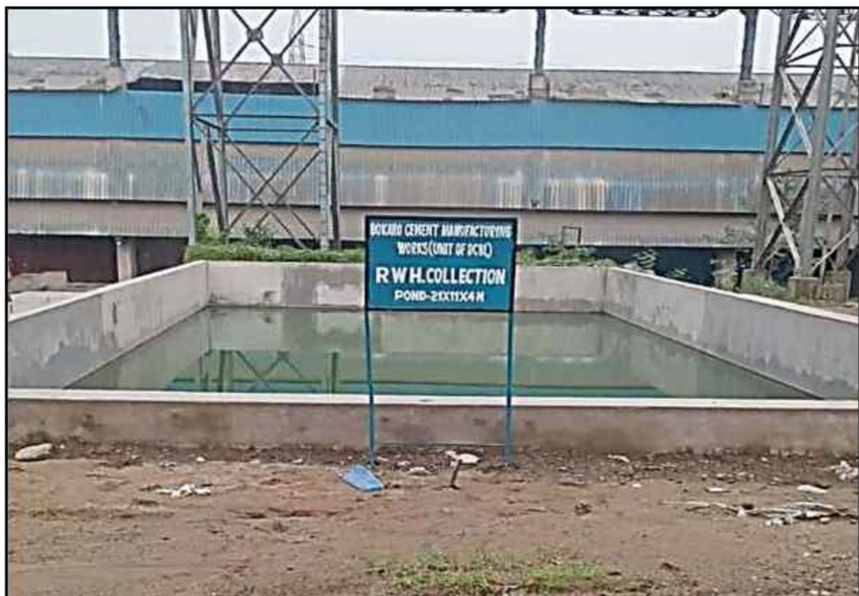
Rain Water collection Pond constructed Capacity: 925 KL
